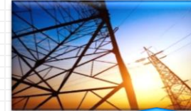
Project: Indo-German Energy Programme – Green Energy Corridors (IGEN-GEC)
